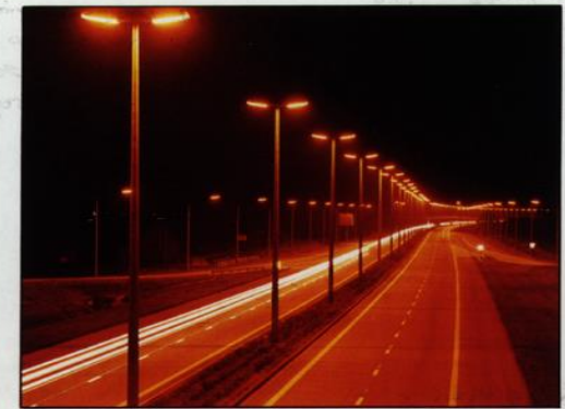
Plate 9 Motorway lighting with low pressure sodium lamps.
