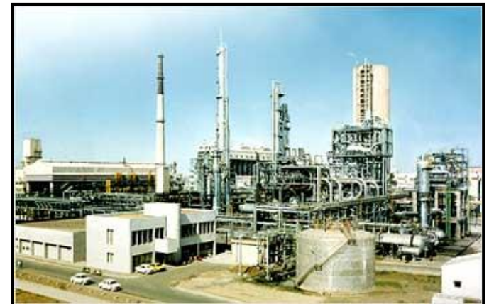
Facility for NH 3 production
