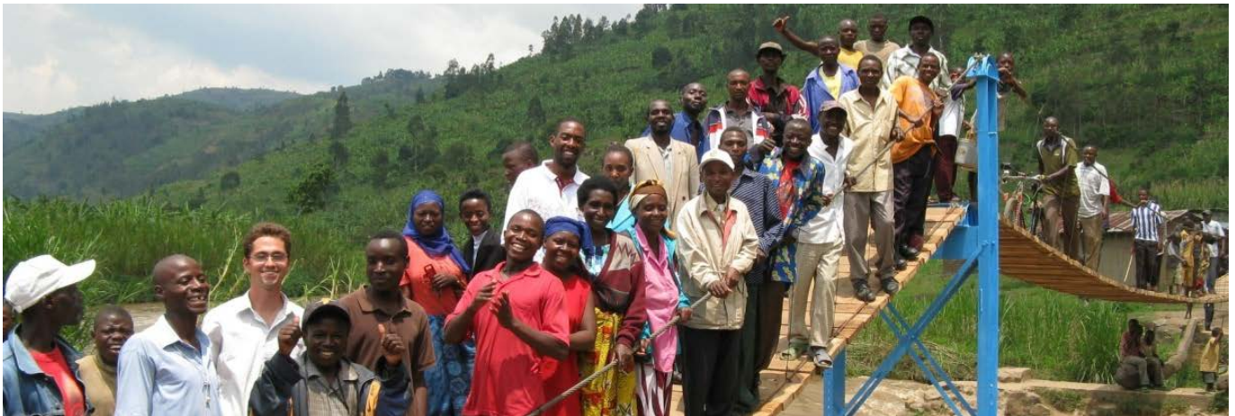
Brückenbau in Nyabarongo, Ruanda
